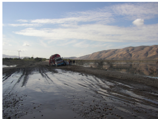
Flooded highway outside of Gonaïves, Haiti
